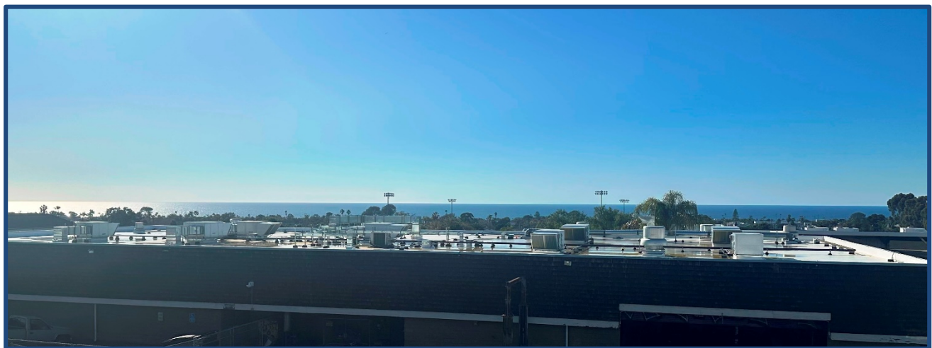
(San Dieguito HS Academy Roof Heating Ventilation Replacement)
